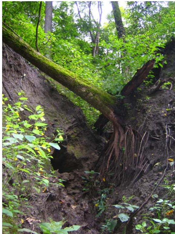
Figure 10. Picture taken just below 345 meter nick point. Walls become steeper at this section, and roots become exposed as root systems fail.
