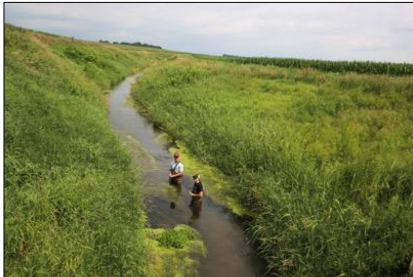
Figure 1. This is an example of an open drainage ditch in south-central Minnesota.
