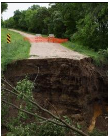
Figure 3. (Above) Road washout in Belle Plaine, MN in 2014. (Ruud, 2014)
