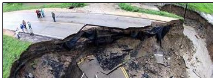
Figure 3. (Above) Road washout in Belle Plaine, MN in 2014. (Ruud, 2014)
