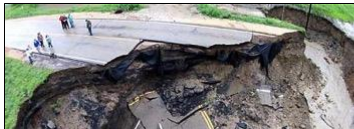
Figure 2. (Above) Road washout in Belle Plaine, MN in 2014. (Ruud, 2014)
