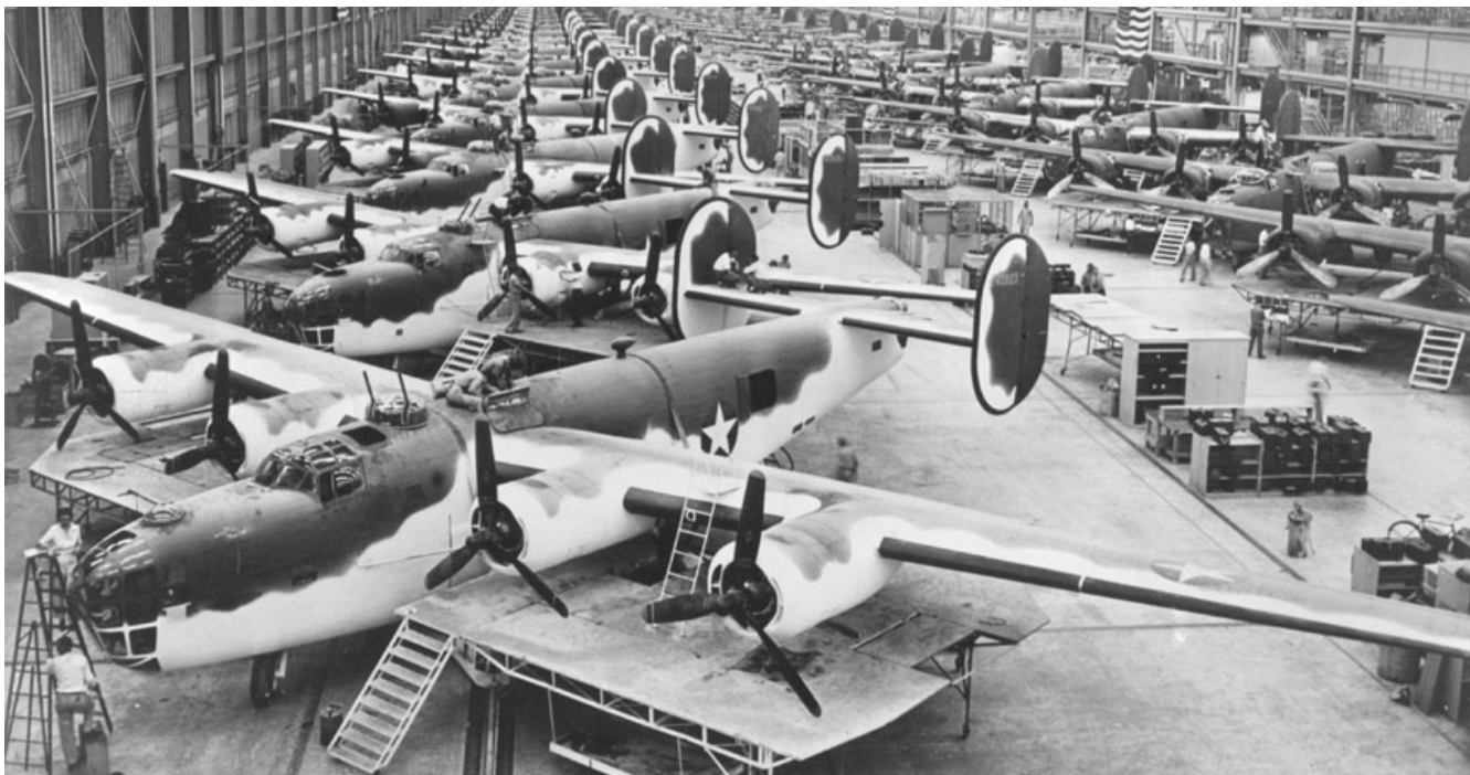
Mass production of Consolidated-Vultee B-24 Liberator heavy bombers at the Consolidated factory in Fort Worth, Texas, in 1943. More than 18,000 B-24s were built between 1940 and 1945.
