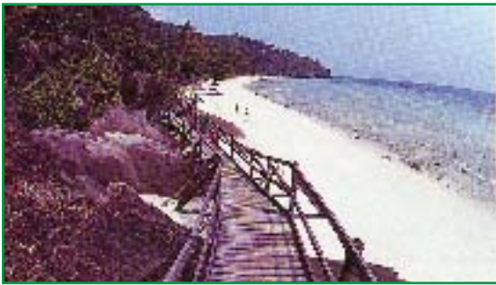
An elevated beach walkway at Pulau Pimang
